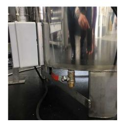
Picture 3. Filling and discharge pipe for heating water
