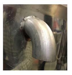
Picture 4. Overflow pipe for heating water
